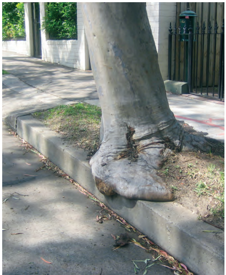
Trees with vigorous root systems may damage road infrastructure.
