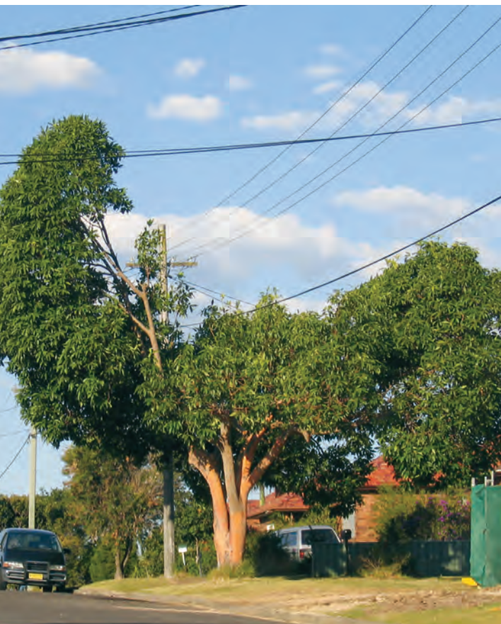
Where trees share the road verge with aerial utility services large trees suffer severe lopping that compromises the trees form and health. Tree selection should consider these constraints.
